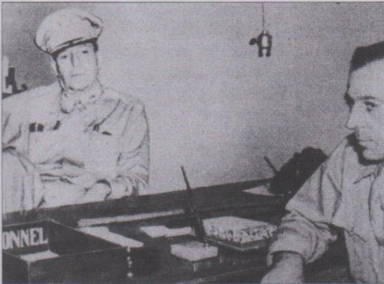
General Douglas MacArthur and Major-General Richard Sutherland in their office in the Malinta Tunnel, March 1, 1942. The tunnel was built as a protected site from aerial bombardment. During the 1942 siege it housed the various command staffs, a hospital, civilians, and supplies for the island's garrison. (US Army, NARA)
