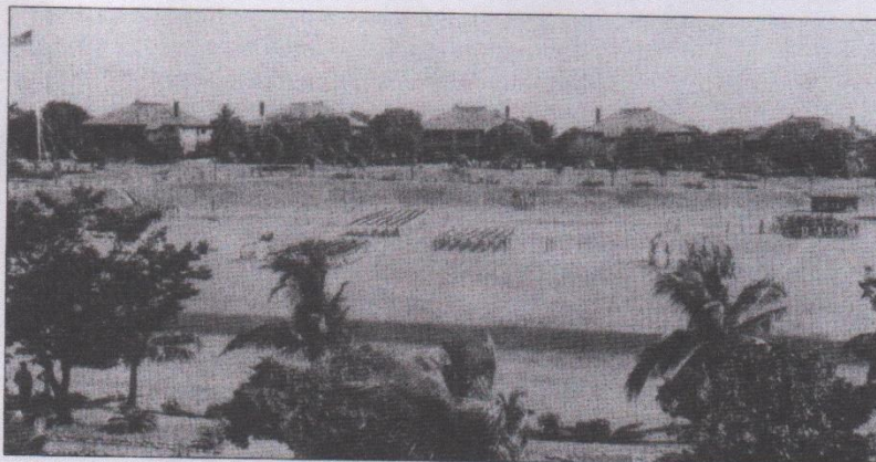
The parade ground, Topside Fort Mills, in the 1930s. The top image is from a series of photographs taken by a non-commissioned CAC officer in 1930 (courtesy of the Karl Schmidt collection). The large building nearest to the flagpole is the Post Headquarter. The bottom image was taken by M.Sgt. Charles Coffin. The buildings in the background are the married officers' quarters.
